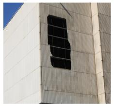
The C-633-4 Cooling Tower located to the east of the C-333 Process Building was also damaged. Large fiberglass shrouds located at the top of the tower were blown off along with some transite and sheet metal panels. Due to the USEC shut-down, the cooling tower was not in operation at the time of the incident.
